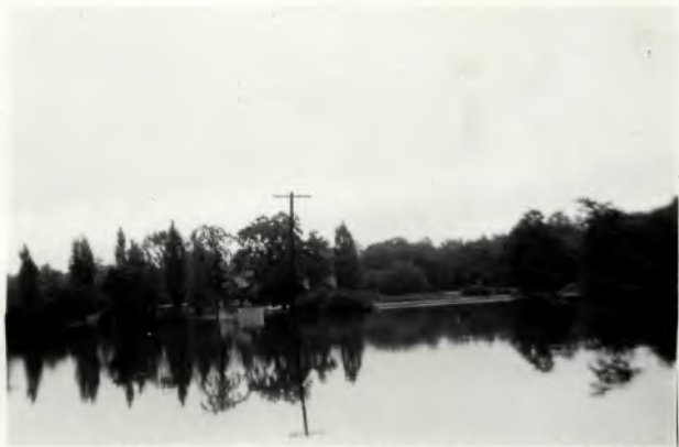
FLOODED DAM No 1 1938
