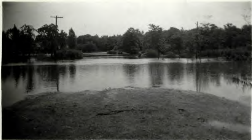
FLOODED ENTRANCE. DAM NO 1
